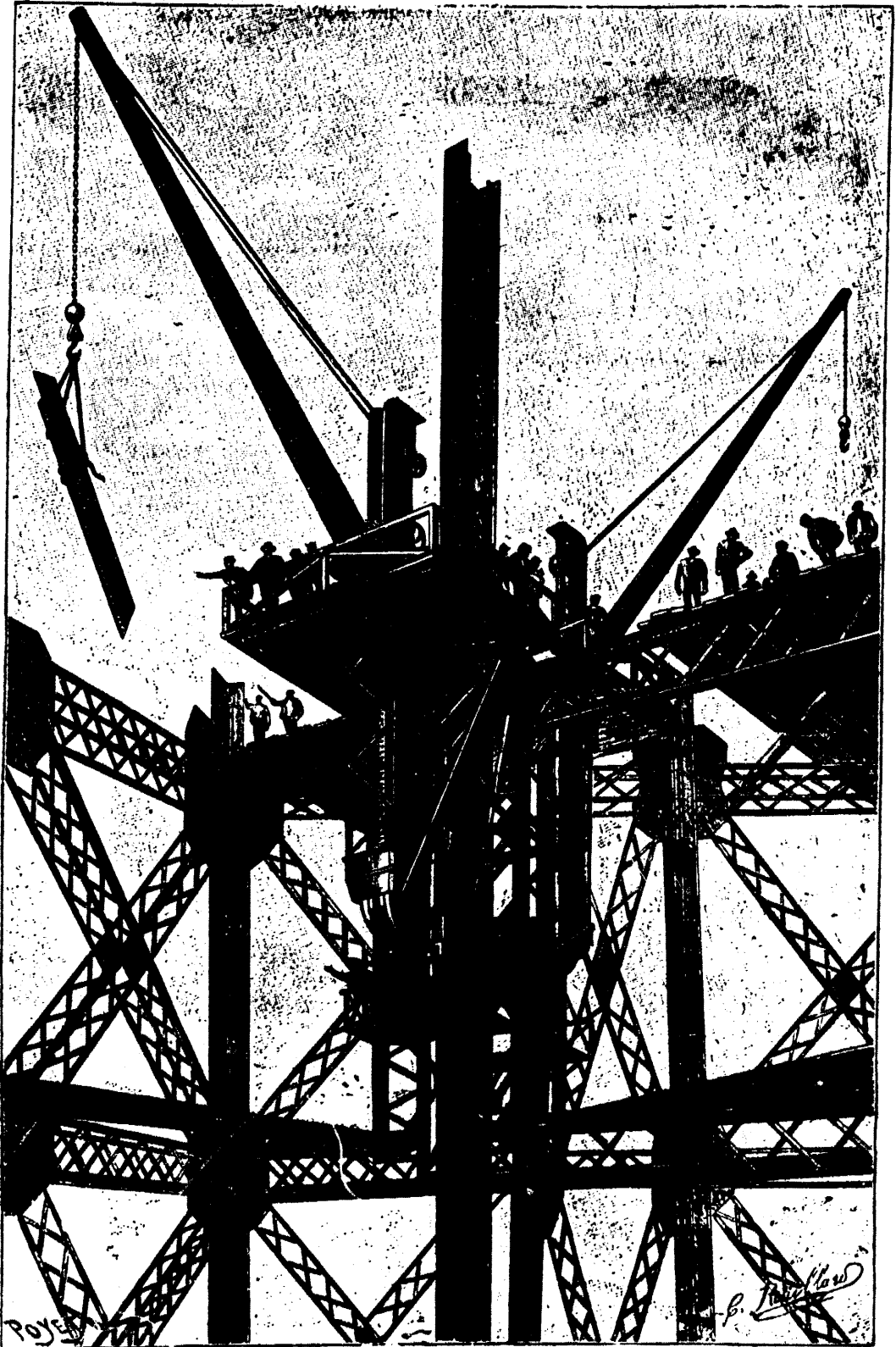
FIG. 239.—Arrangement of the crane for constructing the tower above the second story. Height 215 meters. December, 1888.
