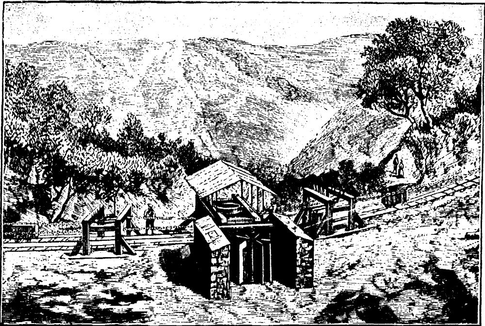
FIG. 51.—Transportation by hanging chains at Aïn-Sedma. Station at head of section.
