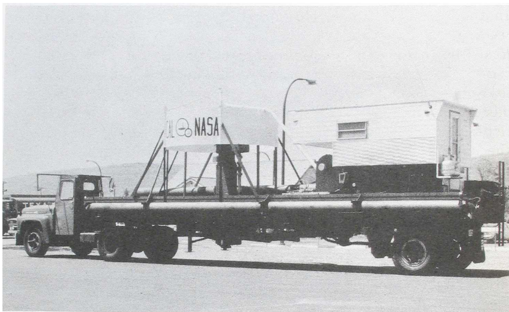
Figure 4-12. Ground-spray equipment for seeding fog.
